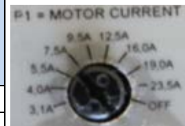
Figure: P1 of a 7.5 kW motor starter
