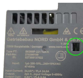
Frequency inverter without STO contact jumper
